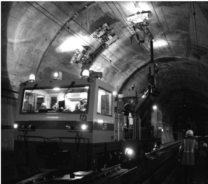
Concrete Lining Inspection Car (CLIC)
