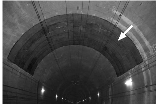
Repaired concrete tunnel
