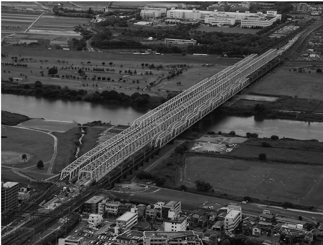
Replacement of Tone River Bridge
