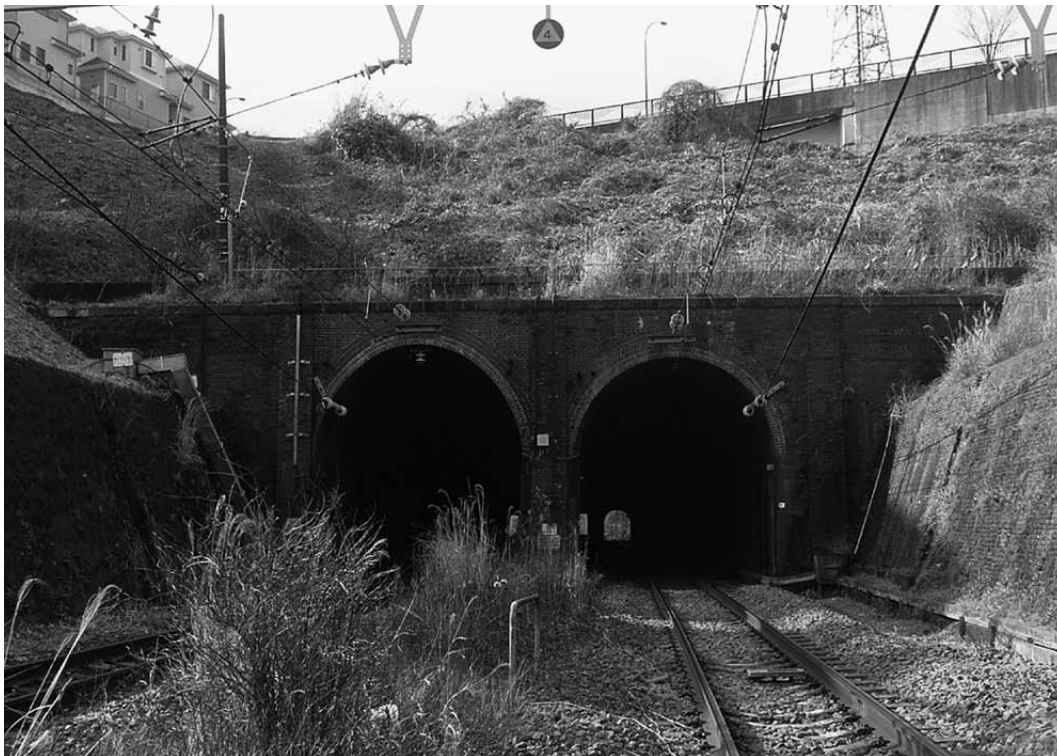
126-year-old Shimizuyato Tunnel
