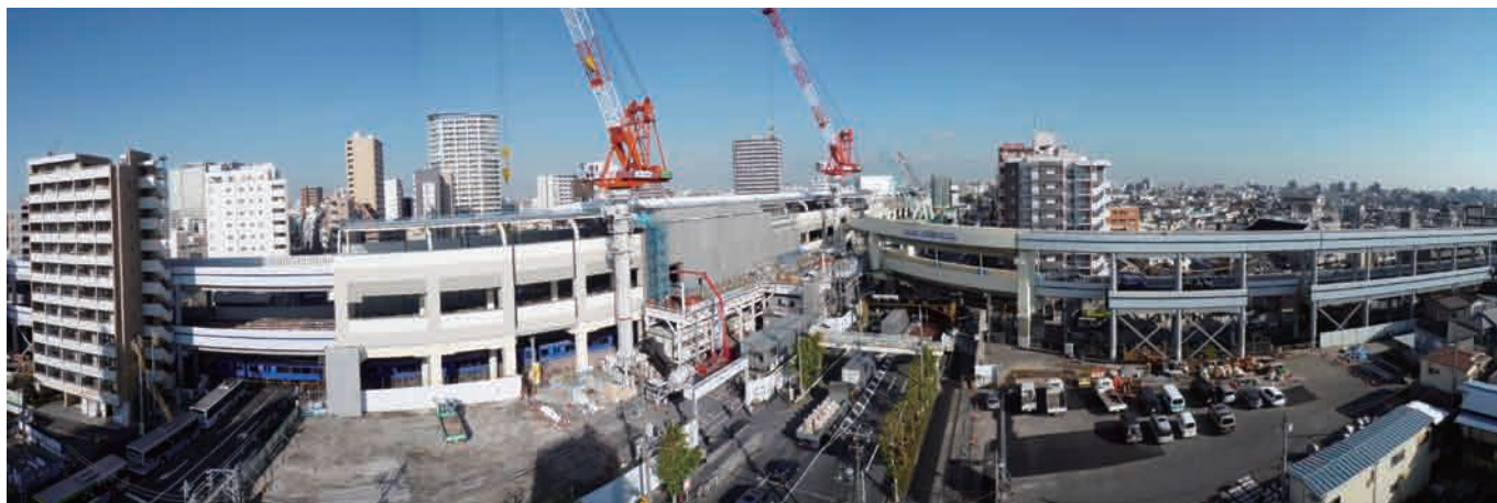
Keikyū Kamata Station under renovation
