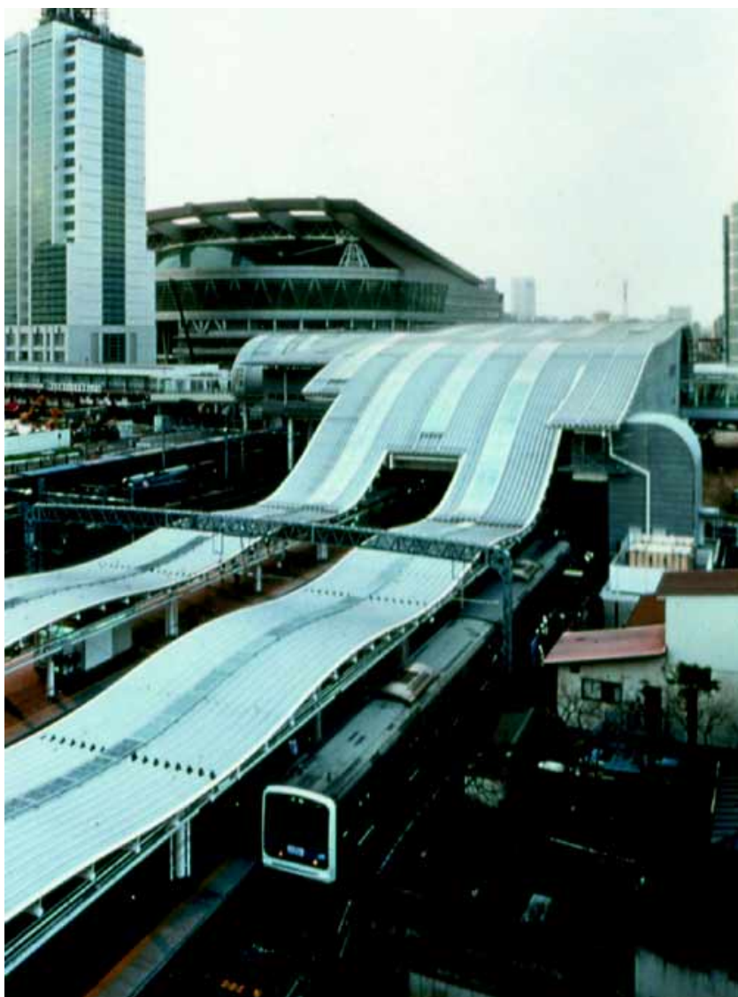
JR East's Saitama Shin Toshin Station on Tohoku main line (2005). Designed by architect Mr Edward Suzuki. (JR East)
