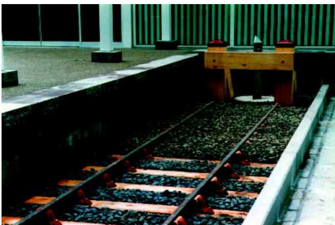
A 7-meter length of the original track has been built using period double-headed rails seated in reproduction chairs on new timber sleepers. The first 4 meters from the wooden buffer and Mile Marker Zero show how the ballast was filled up to the rail heads in the early days. (EJRCF)
