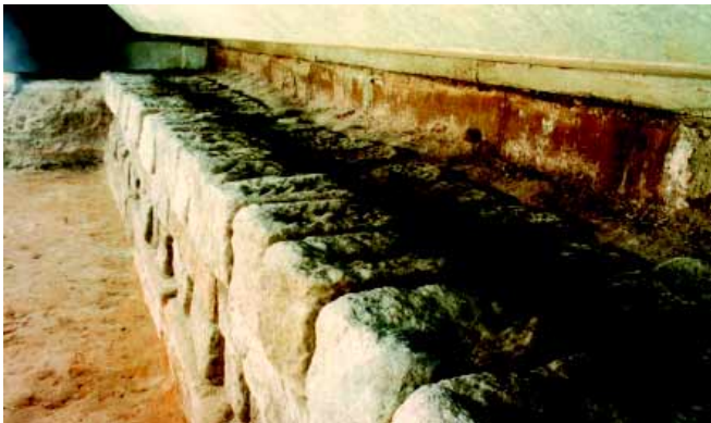
Part of the original station foundations can be seen through a floor window in the newly rebuilt Old Shimbashi Station. (EJRCF)
