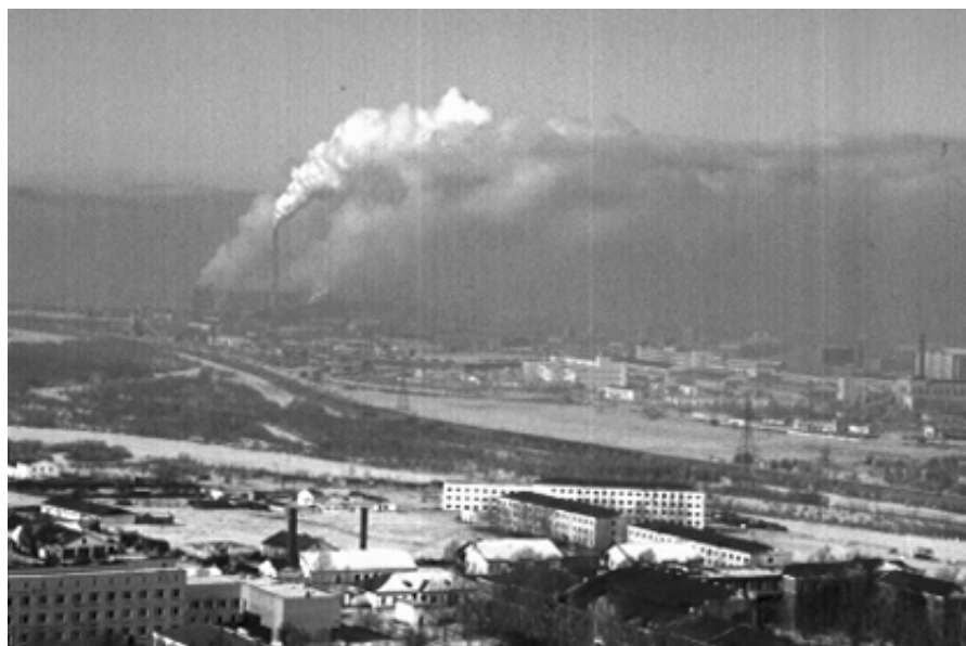
Power station in Ulan Bator, Mongolia
