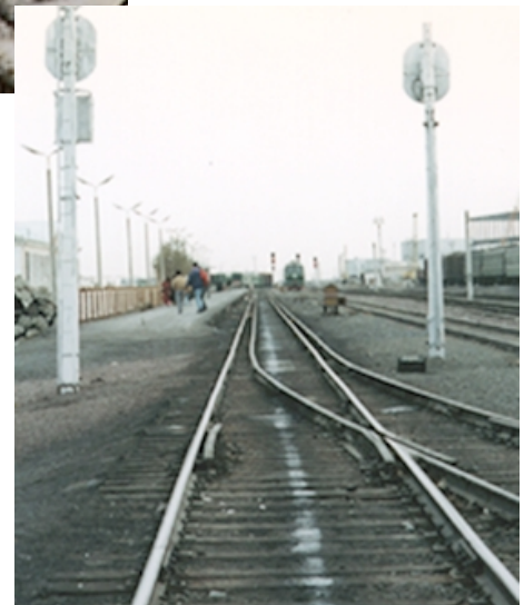
The passenger platform at Druzhba Station, has a four-rail track to receive both Chinese (1435-mm gauge) and Kazakhstani (1520-mm gauge) trains.
