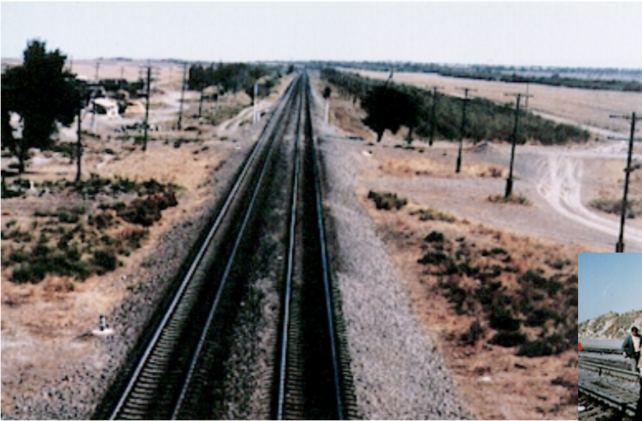
This non-electrified double track in Uzbekistan linking Samarkand with Tashkent is well maintained.
