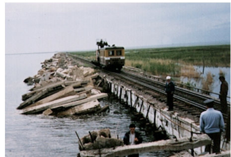
The Aktogay-Druzhba Line running along a lake side. The track is often flooded, and a new diversion line is being planned.
