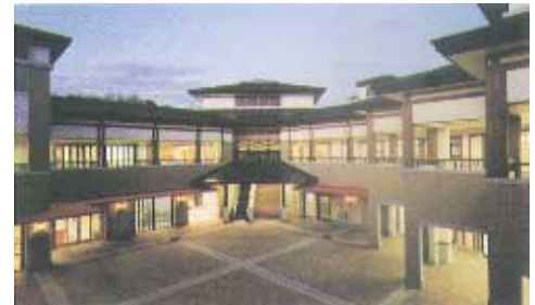
■ Two-storey Shopping Plaza
