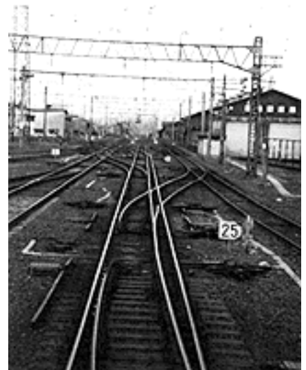
■ Mixed-gauge track is needed between Yamagata and Zao to enable 1067mm freight trains to reach the factories over the lines not used by the Tsubasa Series 400 Mini-Shinkansen. (Author)
